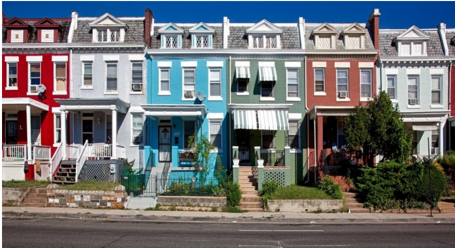
Example 3. Unadapted buildings, with difficult access, main entrance stairs, no ramps and several floors without a lift.
