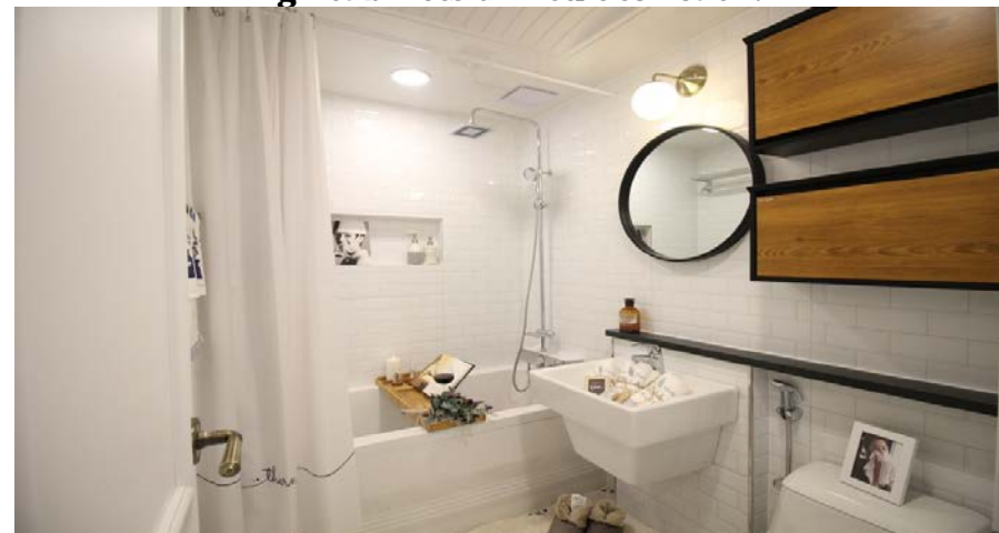
Example 6. Small unadapted bathroom with bath and very high cabinets difficult to reach.
