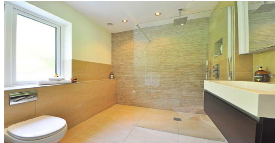
Example 5. Spacious bathroom with walk-in shower and proper lighting, but lacking of several adaptations (bars, shower seats, grab rails, assistant poles, non slip flooring, foldable or fixed seats...)
